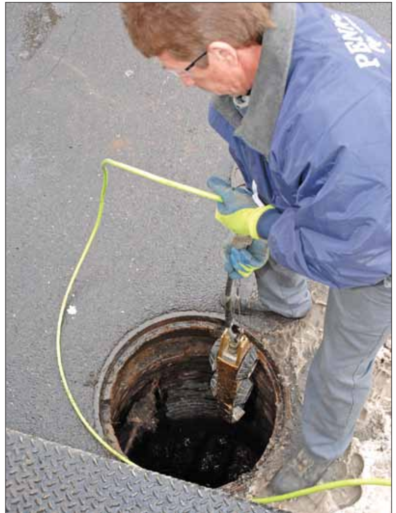
Above: Darryl Stephens deploys a color inspection camera during an inspection demonstration in Trenton, N.J. Below: Supervisor Ray Rios observes an inspection from the company’s TV truck.
