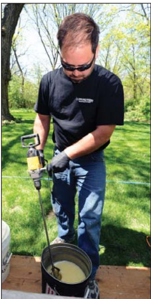
Rickert mixes resin for a CIPP lining job.
