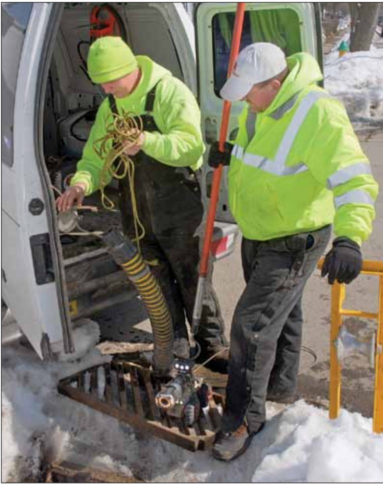
Left photo: Kyle (left) and John Baxter prepare to launch an Aries Pathfinder camera. Right: Kyle monitors an inspection inside the company's camera van from Aries Industries Inc. Equipment includes a Saturn III control unit, a tractor control unit and a laptop computer and auxiliary monitor.
