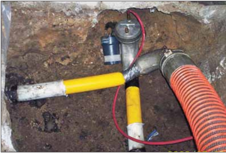
Workers lined in both directions from the access point in the 184-foot-long 4-inch pipe, shooting 101-foot and 83-foot liners.
