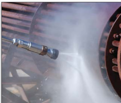
Safe and effective surface preparation.
