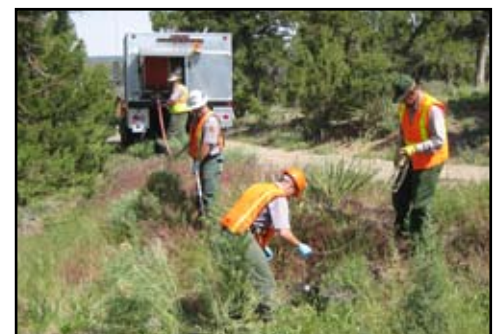
Culvert cleaning the smart and safe way!
