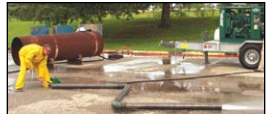
The Badger going through 4" pipe with multiple bends
