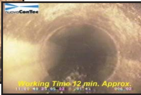
Grease removal from 13.8" line
