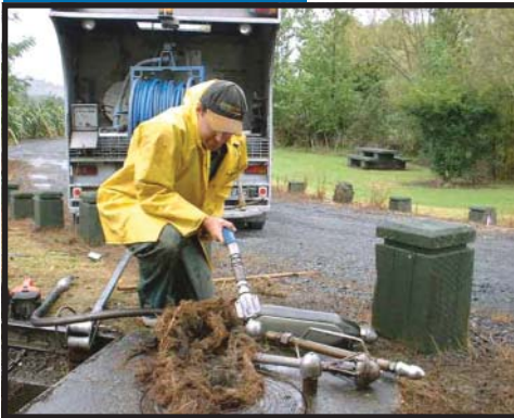
WH-3/4 rescues other nozzles stuck in root mass in New Zealand
