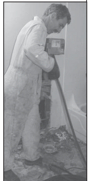
Robert Fulton of Television Inspection Equipment jetting plugged sewer using Warthog.
