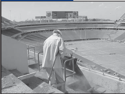
Removal of elastomeric coatings and caulk joints at Buffalo Stadium
